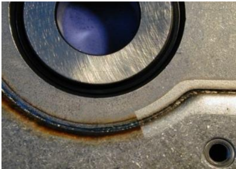
Welding line cleaning
