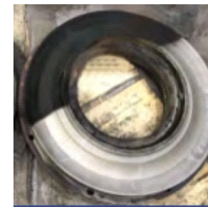
Flange surface coating removal
